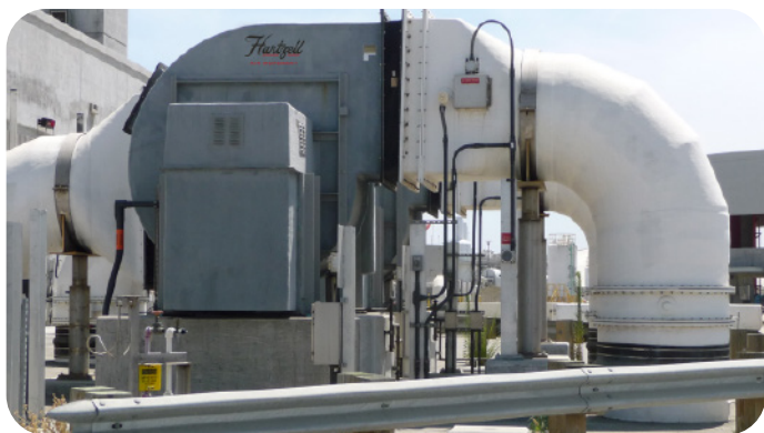
Series 41 Fiberglass Backward Curved Centrifugal Fan, Arrangement 8
