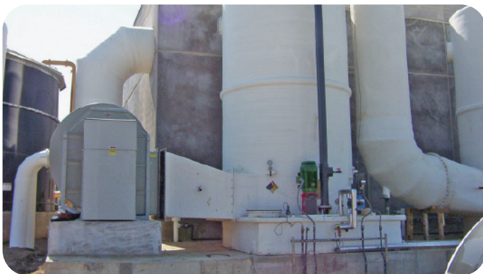
Series 41 Fiberglass Backward Curved Centrifugal Fan with Scrubber
