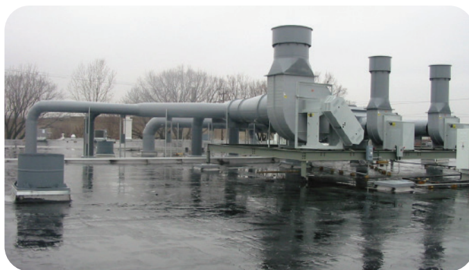
Series 41 Fiberglass Backward Curved Centrifugal Fan with Stack Caps
