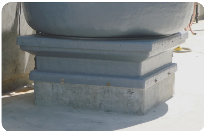
Series 88 Fiberglass Exhauster with Custom FRP Base
